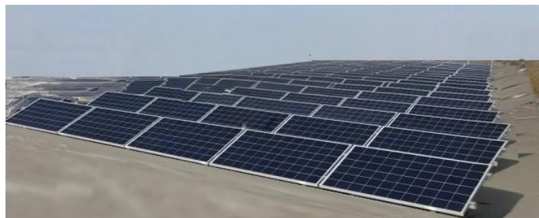
Fig. 5 Example of a modular PV system that can be operated as a tracking PV system with higher efficiency, or as a standard fixed PV system
